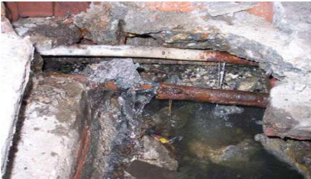
Figure 4. Aged Water Pipe Broken.
