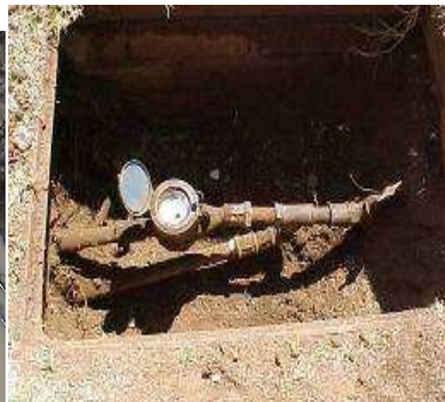
Figure 7. Poor Connections and Meter By-Passing.
