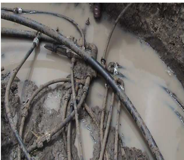
Figure 7. Poor Connections and Meter By-Passing.
