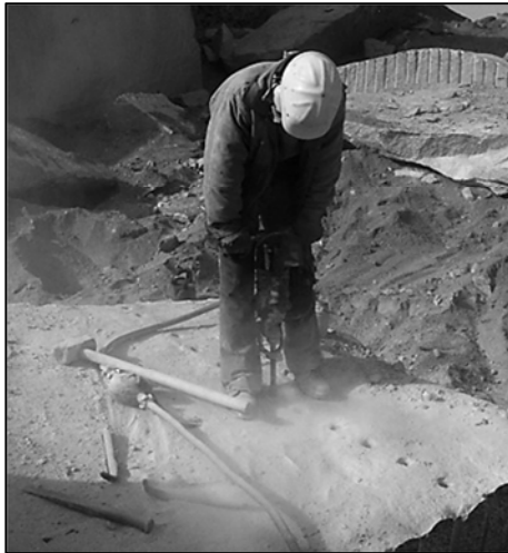
(a) Drilling of a rock block.
