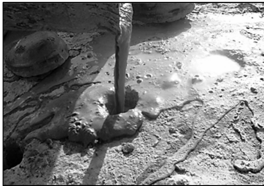
(b) Pouring of the NEEM into the holes.
