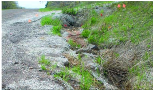
Figure 2. Unstable ditch. Source (Faisca et al., 2012).
