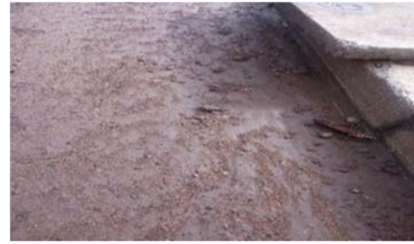
Figure 13. Sedimentation of road surface and drainage structure
