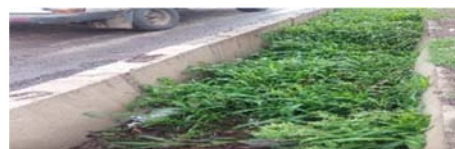
Figure 10. Plants grown in drainage structure, photo.
