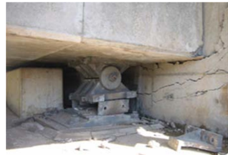
Figure 2. Damage of movable bearing of Imokawa Bridge due to collision.
