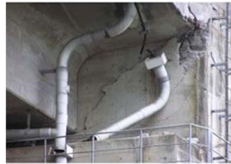
Figure 1. Damage of parapet wall of Imokawa Bridge due to collision.
