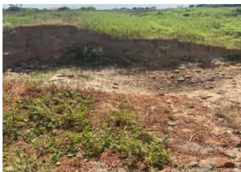
Figure 11. Rupture at the spillway.
