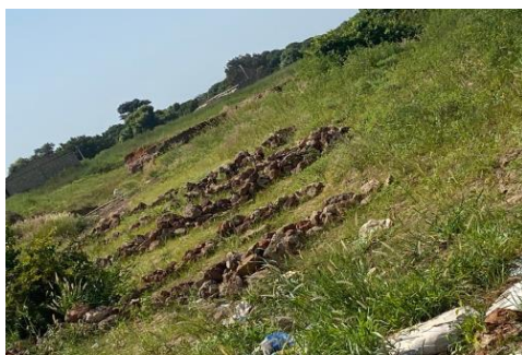
Figure 9. Rows of rocks to reduce wave pressure.
