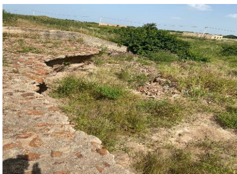
Figure 10. Rupture at the down stream slop.
