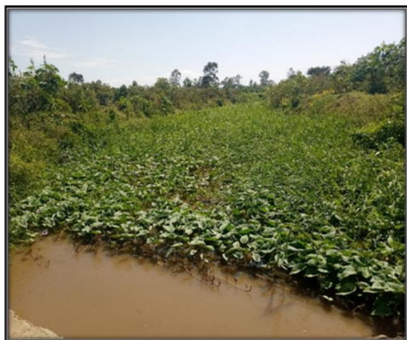
Figure 3. Poorly maintained irrigation canal invaded with aquatic weeds.
