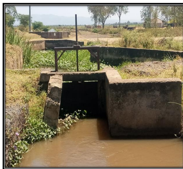
Figure 4. Failing water control structure – Division box.
