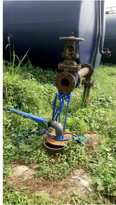
Figure 14. Borehole converted and put into use by a Gas Company operating within the premises.
