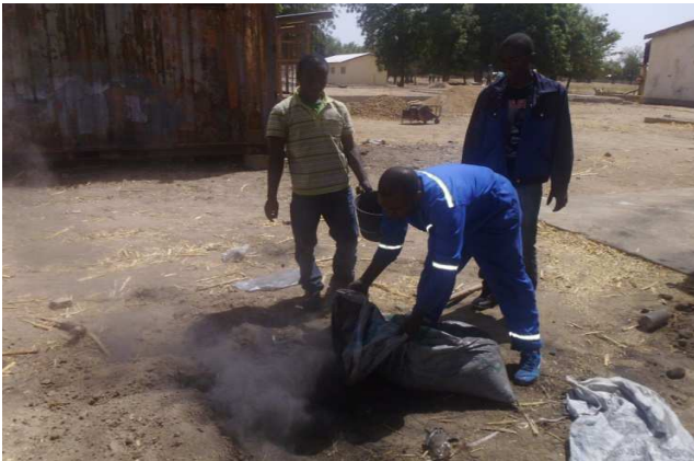
Figure 6. Soil in Grounded portion replaced with biochar.
