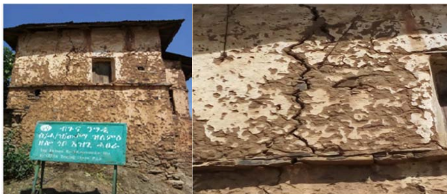
Figure 12. Vertical cracks of Ato Weldegebriel building (by the author).
