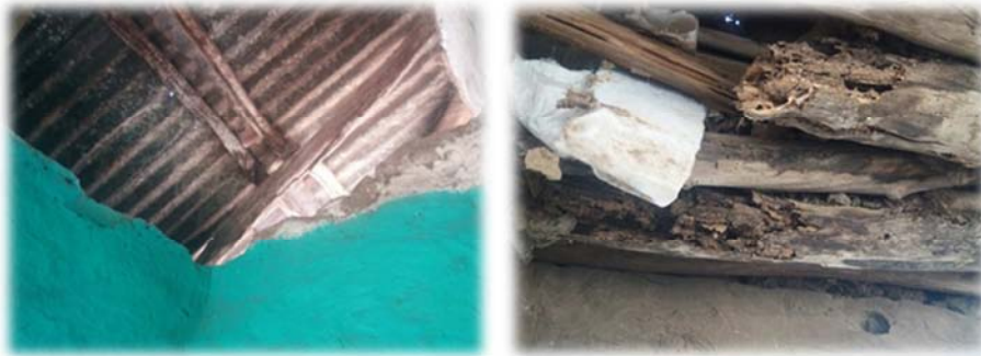
Figure 18. The deteriorated wooden beams and ceilings (by the author).
