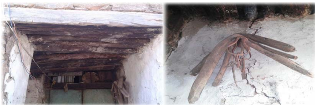
Figure 7. Deteriorated floor and cracked wall (by the author).
