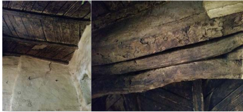
Figure 13. Cracked wall and the deteriorated wooden beam and ceiling.
