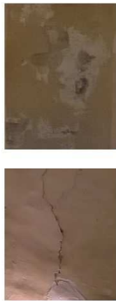
Figure 4. In these pictures, it is possible to recognize the detachments and the lesion visible in the internal part of the church, corresponding to the area in which the GPR survey is acquired.
