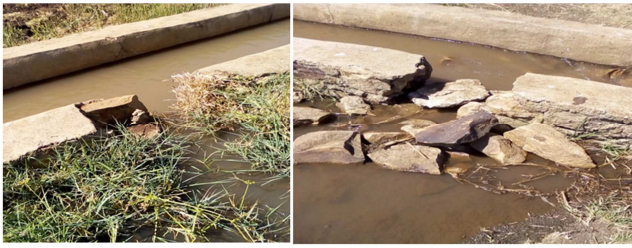
Figure 5. Broken secondary canals and water wastage (losses) in the irrigation scheme.
