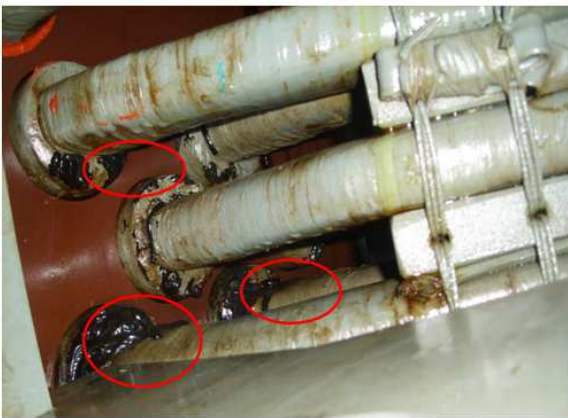
Figure 1. Compound melting due to overheating.
