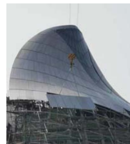
Figure 4. Stainless steel color difference (shady face).
