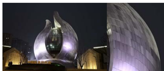
Figure 19. Stainless steel color difference under cold light at night.
