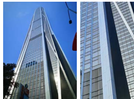
Figure 26. Stainless steel facade of Shenzhen Ping An Centre (effect of six months of natural passivation after cleaning).
