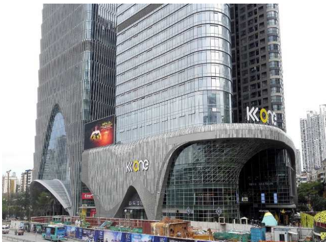
Figure 23. Stainless steel color difference of kkone Shopping Plaza in Shenzhen Binhe Shidai (daytime).
