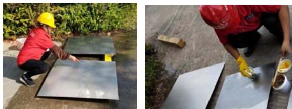
Figure 11. Pickling on outer surface of stainless steel.
