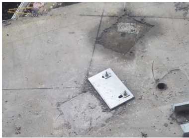
Figure 4. Setting-out of finished surface for curtain wall installation.
