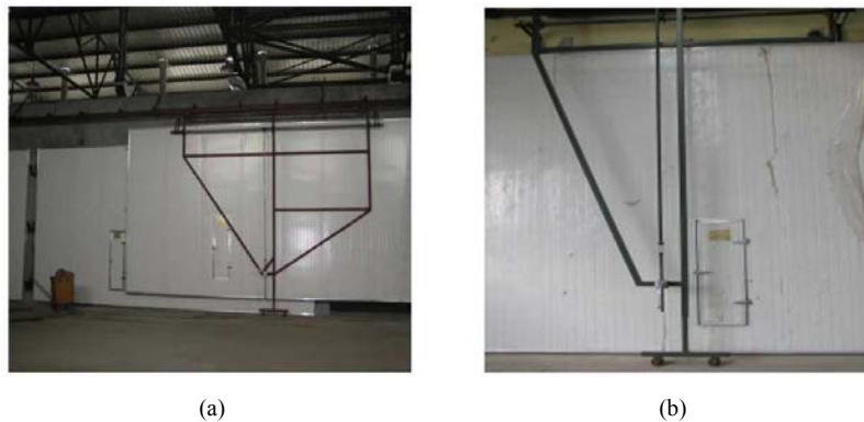
Figure 1. Hand-operated gate lifting device of ordinary drying room.
