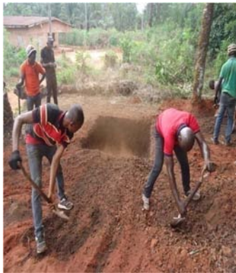
Figure 25. Covering of the trench.
