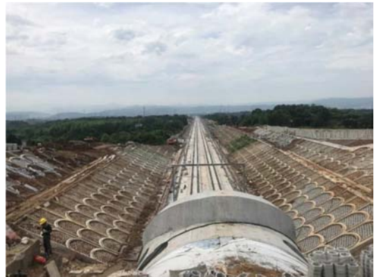
Figure 23. track have been lay on diatomite subgrade.
