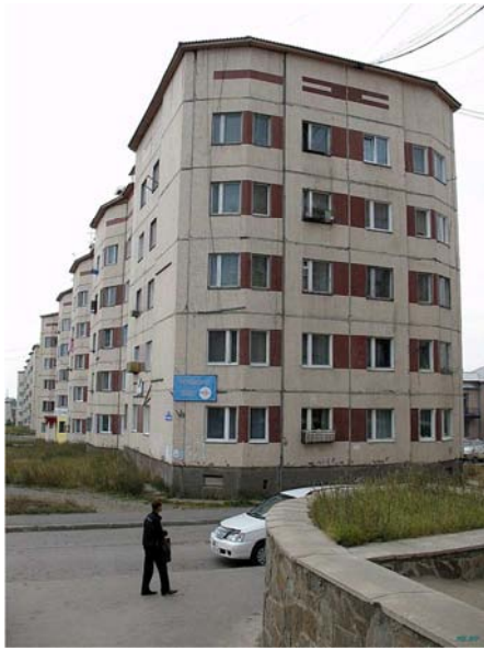
Figure 7. Adaptive seismic protection system by Ya. M. Eisenberg: a) general scheme of seismic protection system: 1 – bearing racks of the ground floor; 2 – connection panels; b) the facade of 122 series building in Severobaykalsk, where an adaptive seismic protection system is used.
