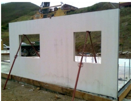
Figure 3. Erection of GFRG panels over plinth beam at site [9].
