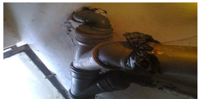
Figure 4. Leakage on main track (soil pipe).
