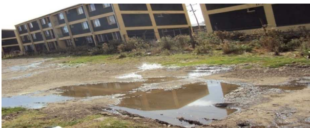
Figure 7. Leakage and over flow of sewage from septic tanks.
