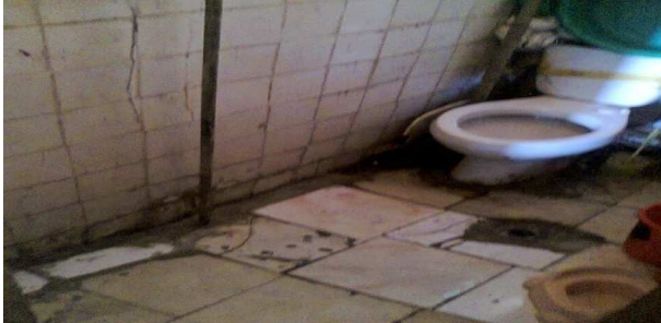
Figure 5. Missed shower tray from construction.
