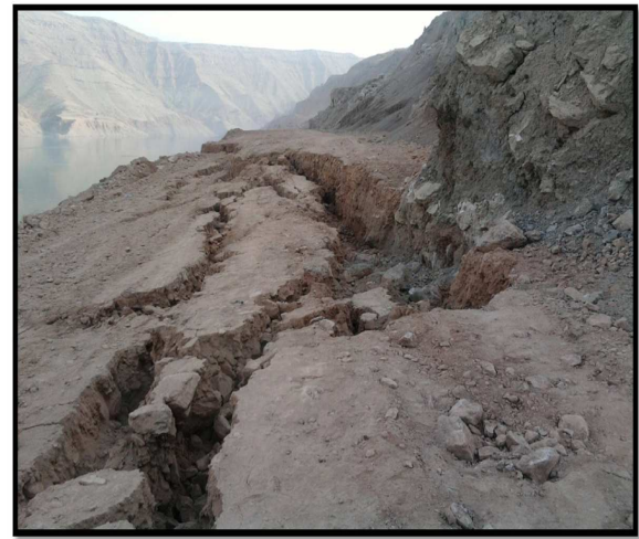
Fig. 3. cracking in the embankment after dam impounding.
