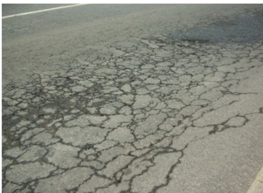
Figure 2. Extensive alligator cracks in wearing course.
