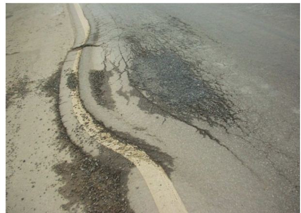
Figure 5. Structural failure and shoving of outer edge of surface course.
