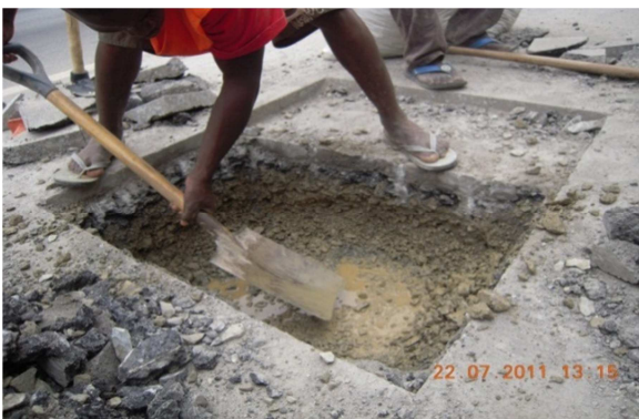
Figure 6. Trial pit showing water-soaked crushed stone base.
