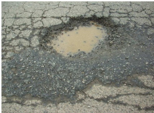
Figure 1. Alligator cracks with pothole development.
