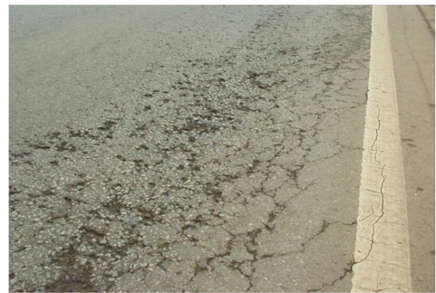
Figure 4. Ravelling with incipient pothole development.
