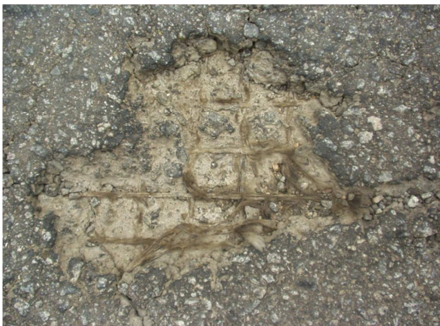
Figure 13. Exposed geotextile placed in an earlier maintenance intervention with thin cover.
