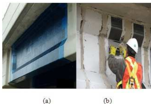
Figure 1. Shear strengthening of Reinforced concrete using CFRP laminate
