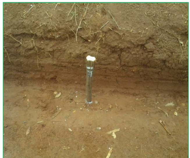
Figure 2. Peg placement at 0+500 on Kuywa-Kopsiro Road.
