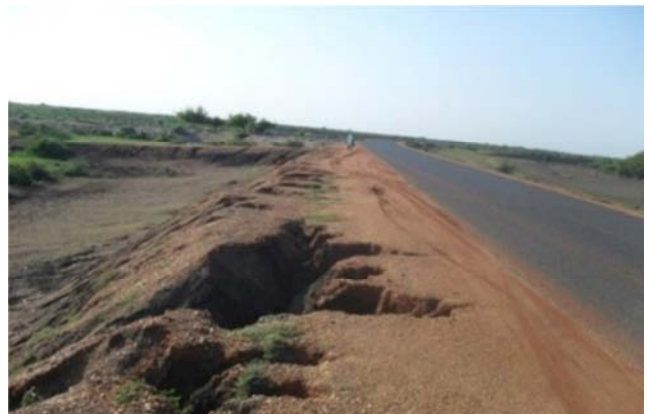
Figure 2. Eroded Al Hosh Slope shows slope situation.
