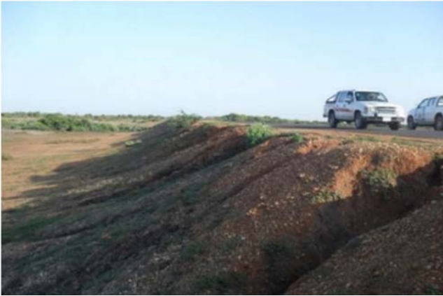
Figure 3. Erosion in Al Hosh Road Slope- left side.
