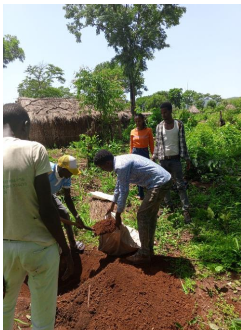
Figure 5. Preparation of soil for mud brick production at site1.
