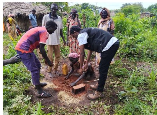
Figure 11. Exposing the mud brick to sunlight.
