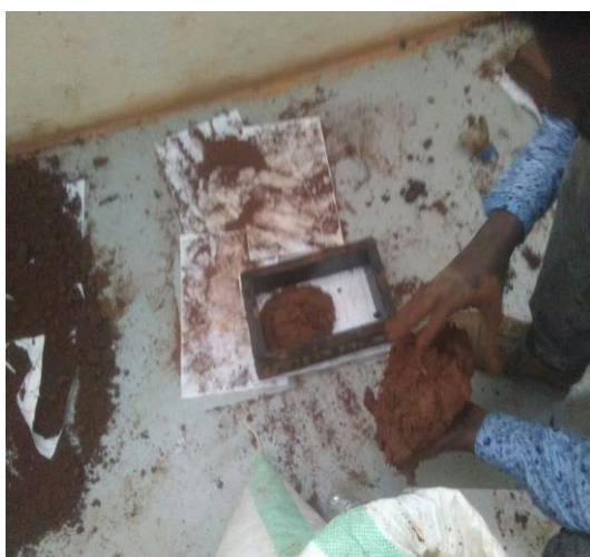
Figure 9. Casting the mud using the Mold.
