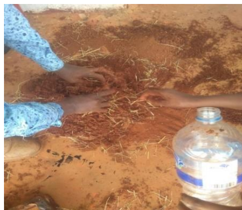
Figure 6. Mixing the soil and the straw at the site.
