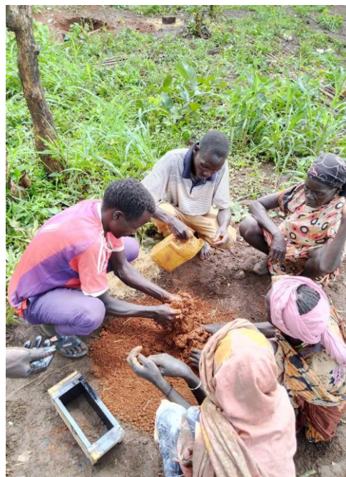
Figure 7. Mixing the soil and the straw with water the site.
