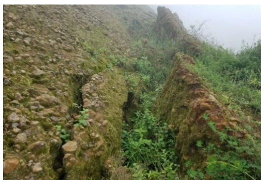
Figure 14. Tension cracks seen between km 32+275 and 32+280.
