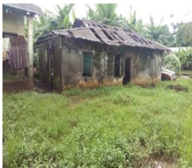
Figure 7. Dilapidated Corrugated Sheet for Building at Grand Hanger and Mabanda Neighbourhoods.
