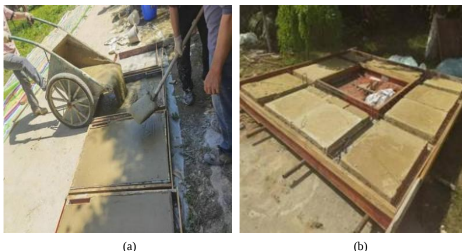
Figure 4. The cement-based porous thermal insulation soil core (a) Production, (b) Installation.
