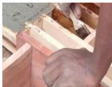
Figure 2. Oiling of the molds.
