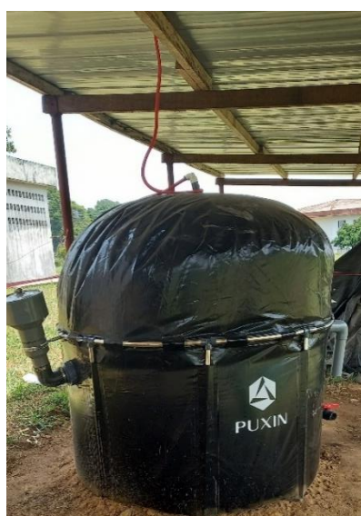
Figure 2. Puxin biogas system.
