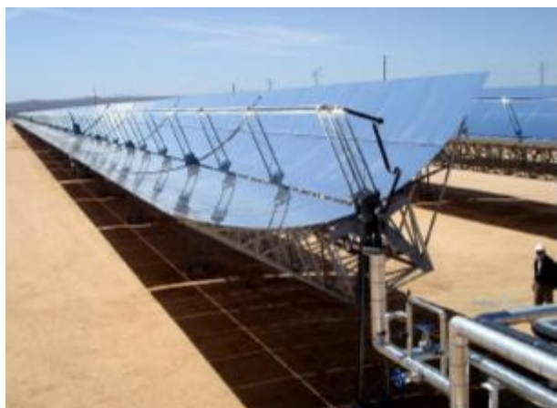
Figure 4. Parabolic trough solar concentrator.
