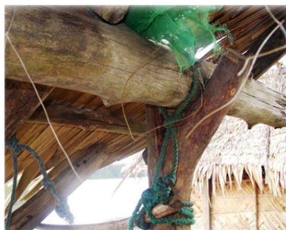
Figure 12. The main Y-shaped timber post ( ikoki ).
