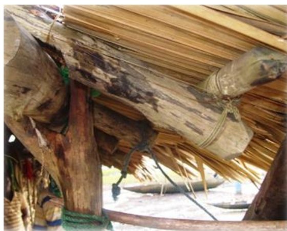
Figure 13. Beam ( som ), rafter ( bamea ) and purlins.
