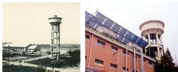
Figure 2. Old Photos and Current Status of the Water Tower.
