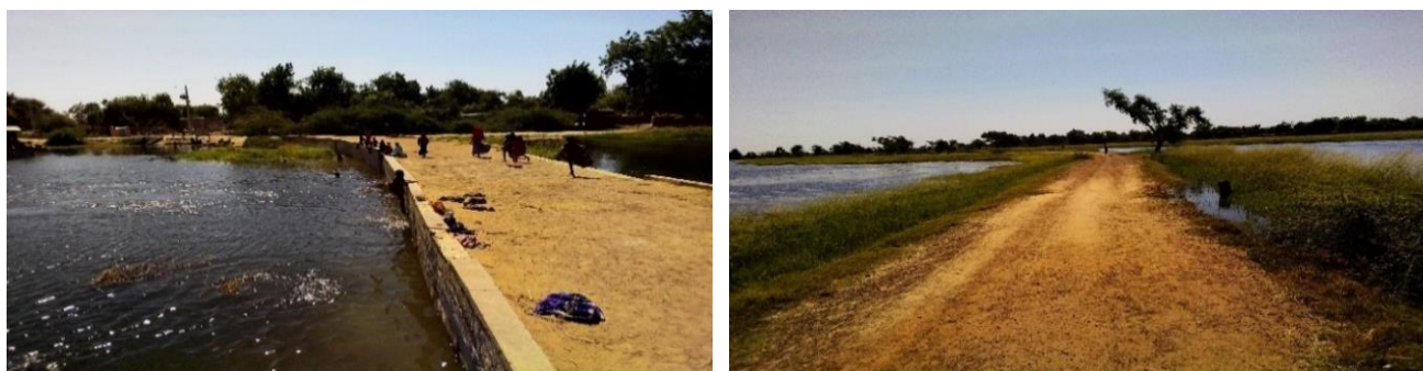
Figure 3. Construction of a dam and dike at LADA, Diffa commune.
