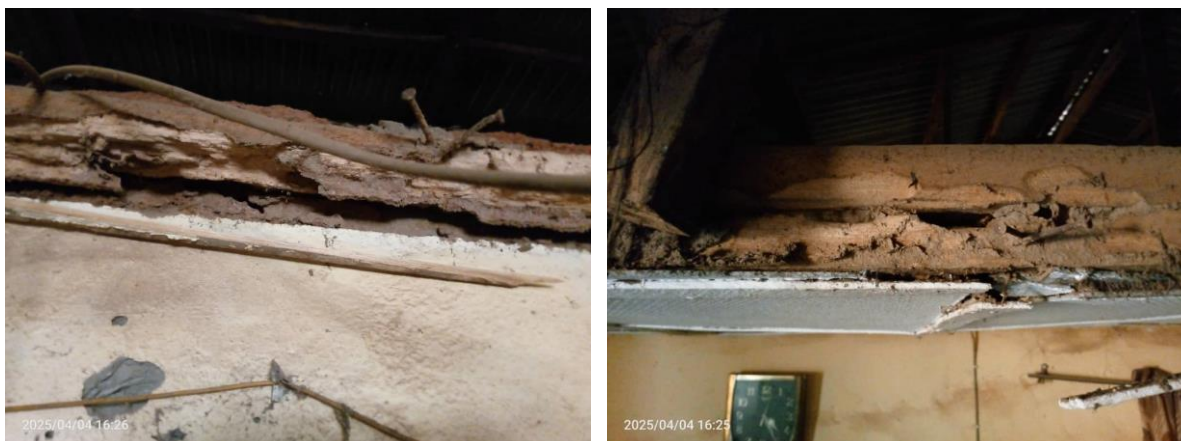
Figure 8. Termite damaged ceiling in a residential apartment in Otukpo.
