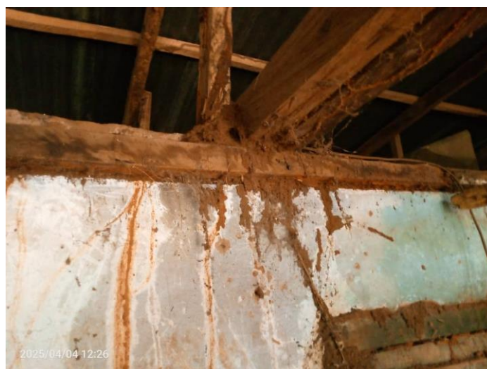
Figure 9. Collapsed ceiling in a residential apartment in Ogbadigbo.
